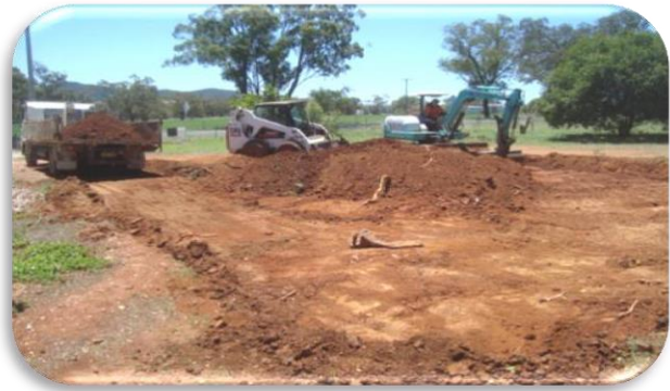
SHED SITE BEING EXCAVATED
