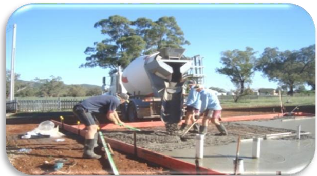
CONCRETE BEING POURED
